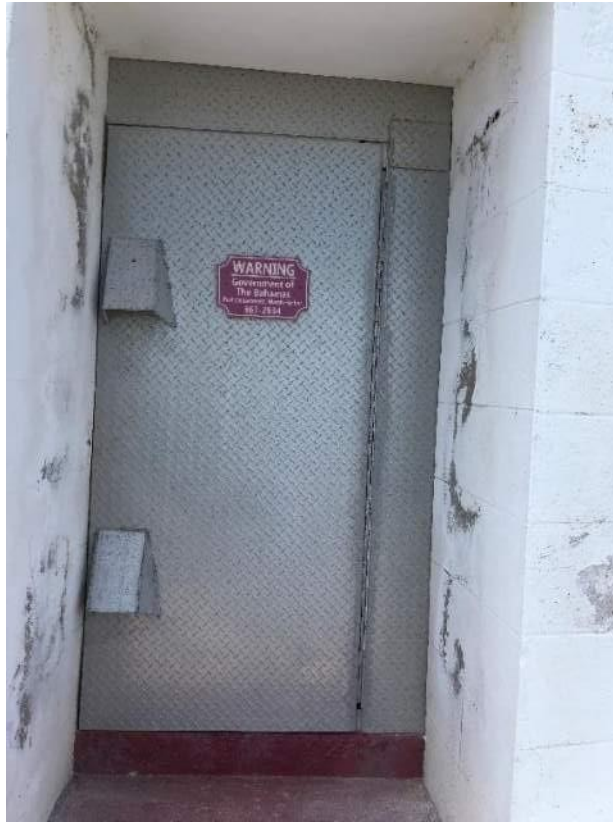
Figure 106. Signage on the entrance at Hole in the Wall Lighthouse.
