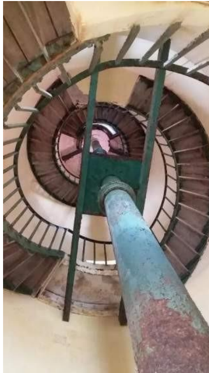
Figure 113. Interior view of Hole in The Wall Lighthouse steel staircase.
