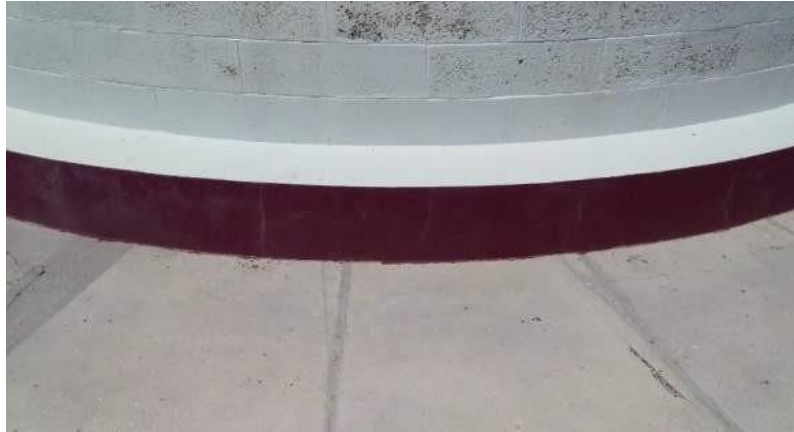
Figure 112. Ground view of Hole in the Wall Lighthouse footing.
